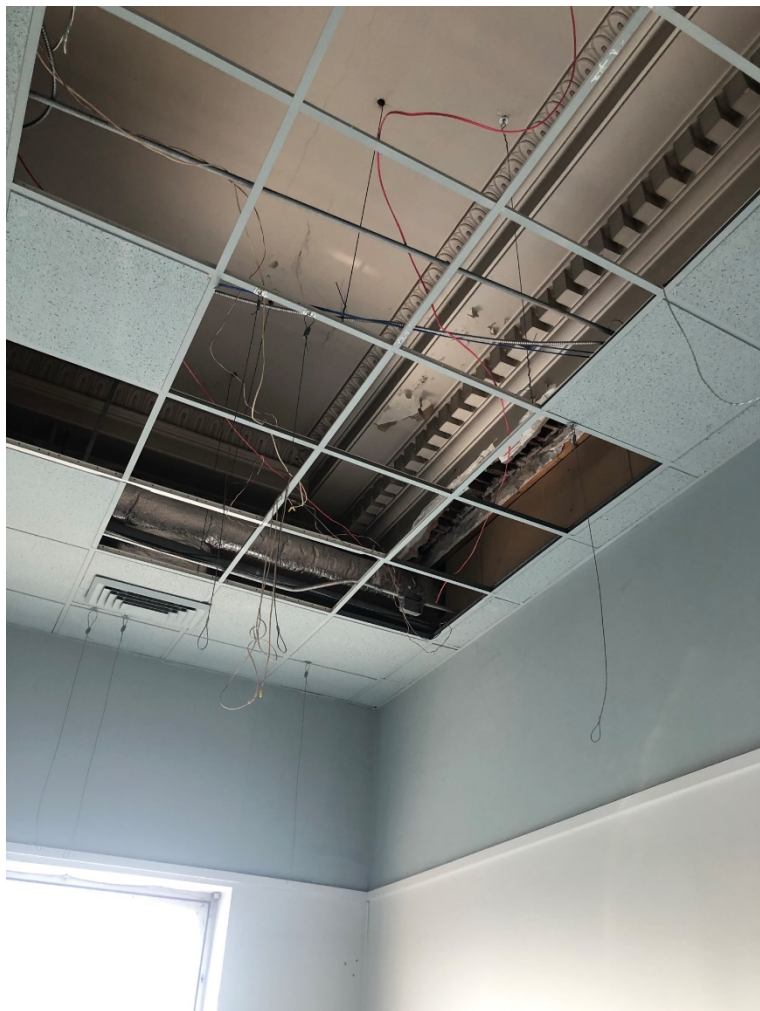
Photo OCH - 3 - 5: Room east of rotunda. Dropped ceiling covers original plaster ceiling. Windows are replacement and openings are partially blocked. Same room as Photos OCH-3-3 through OCH-3-6.
