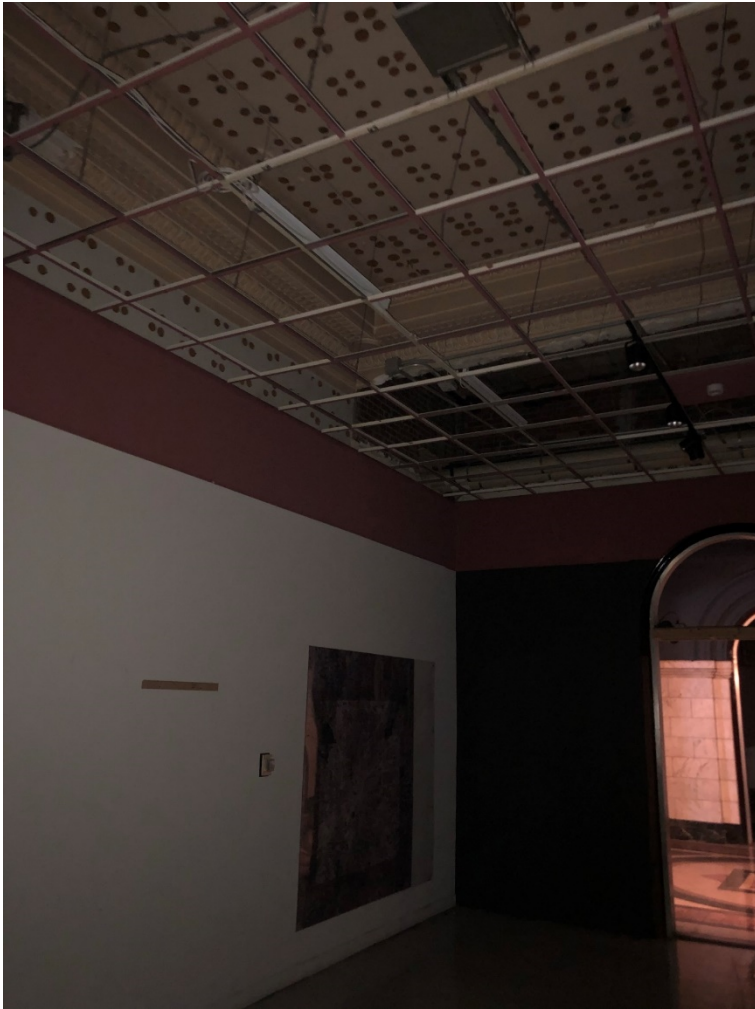
Photo OCH - 1 - 17: Room west of south lobby. Dropped ceiling grid in place. South lobby viewed beyond.
