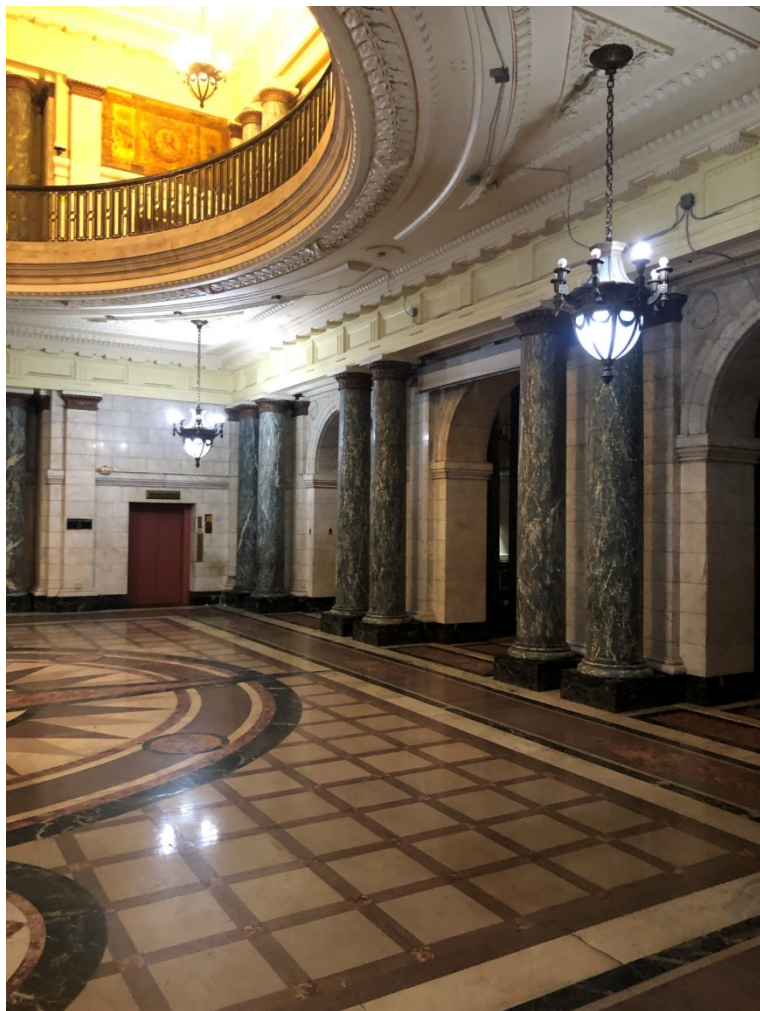
Photo OCH - 1 - 5: Rotunda viewed from north end. Electrical conduits and metal wrapped wiring surface mounted on original plaster and marble.
