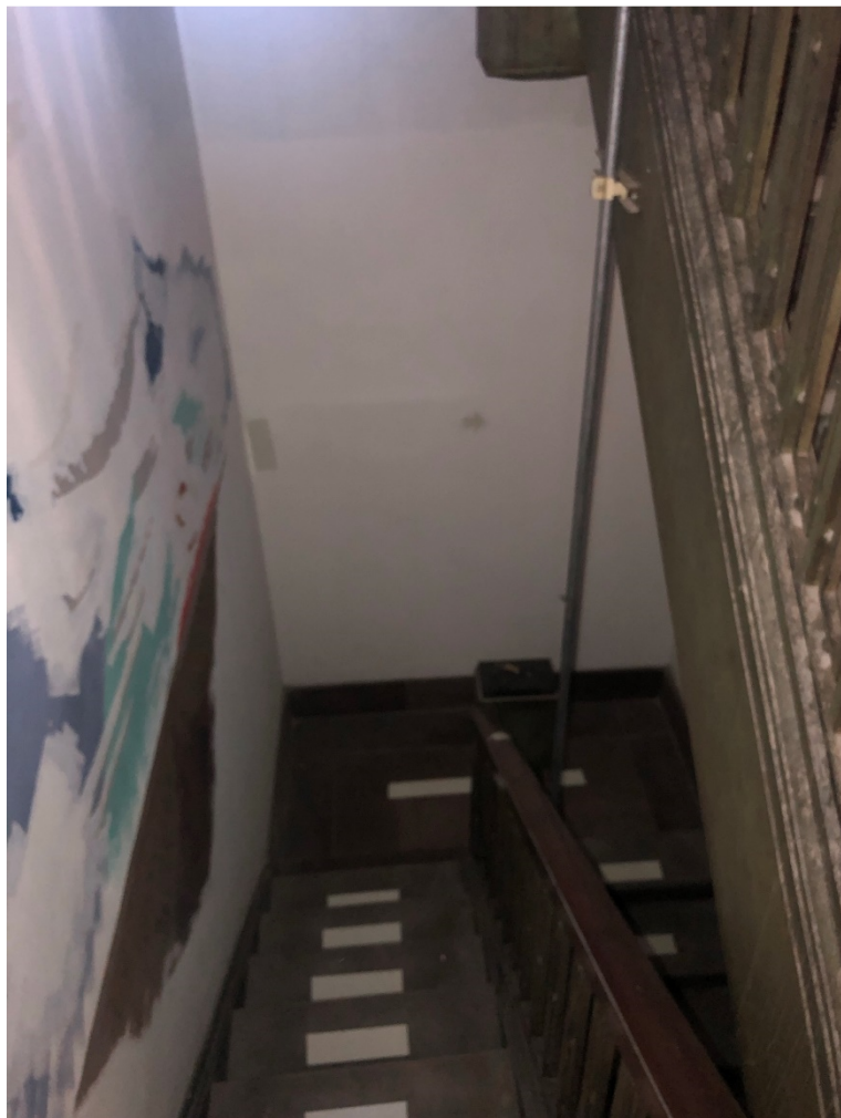
Photo OCH - 3 - 1: North private stair view from 3 rd floor. Handrail only on one side.
