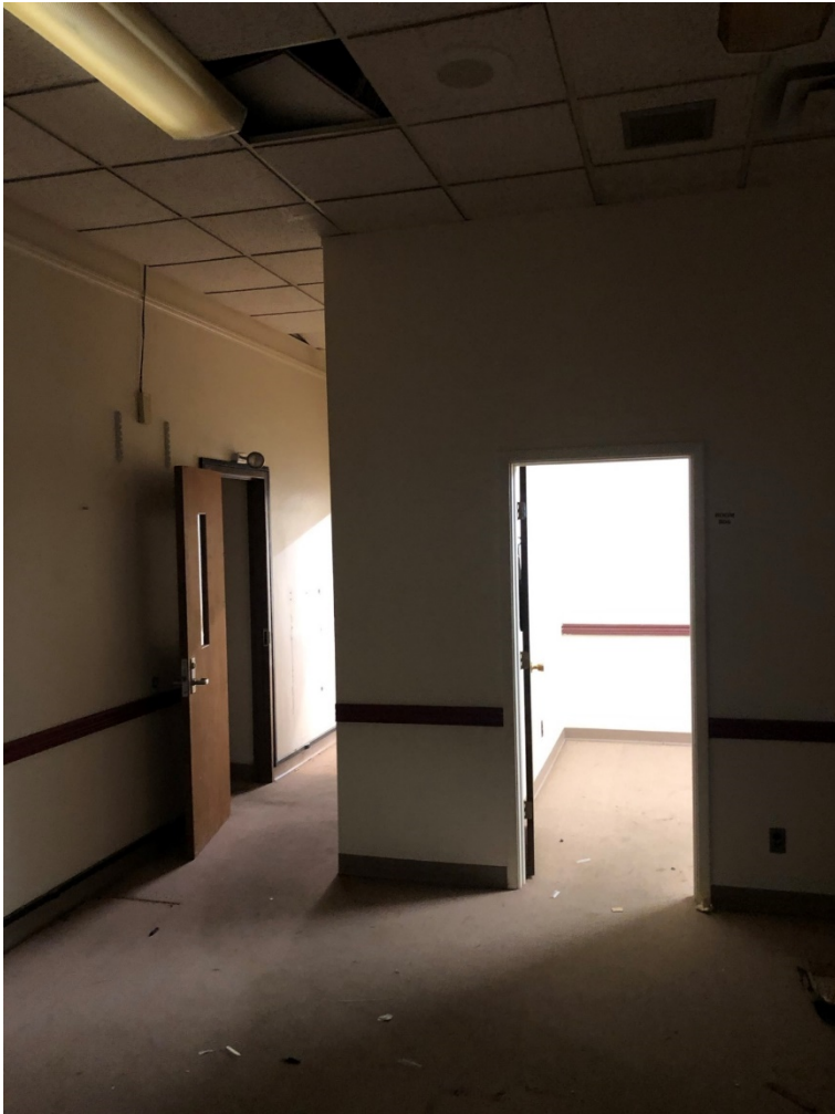
Photo OCH - B - 3: Room west of south lobby. Drop ceiling covers original ceiling. Office partitions are not original.
