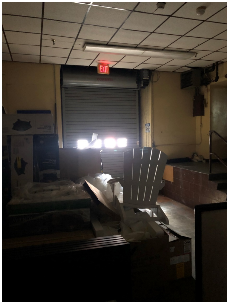
Photo OCH - 1 - 6: Room west of north lobby. Overhead door opens to alley. Dropped ceiling covers original plaster wall.
