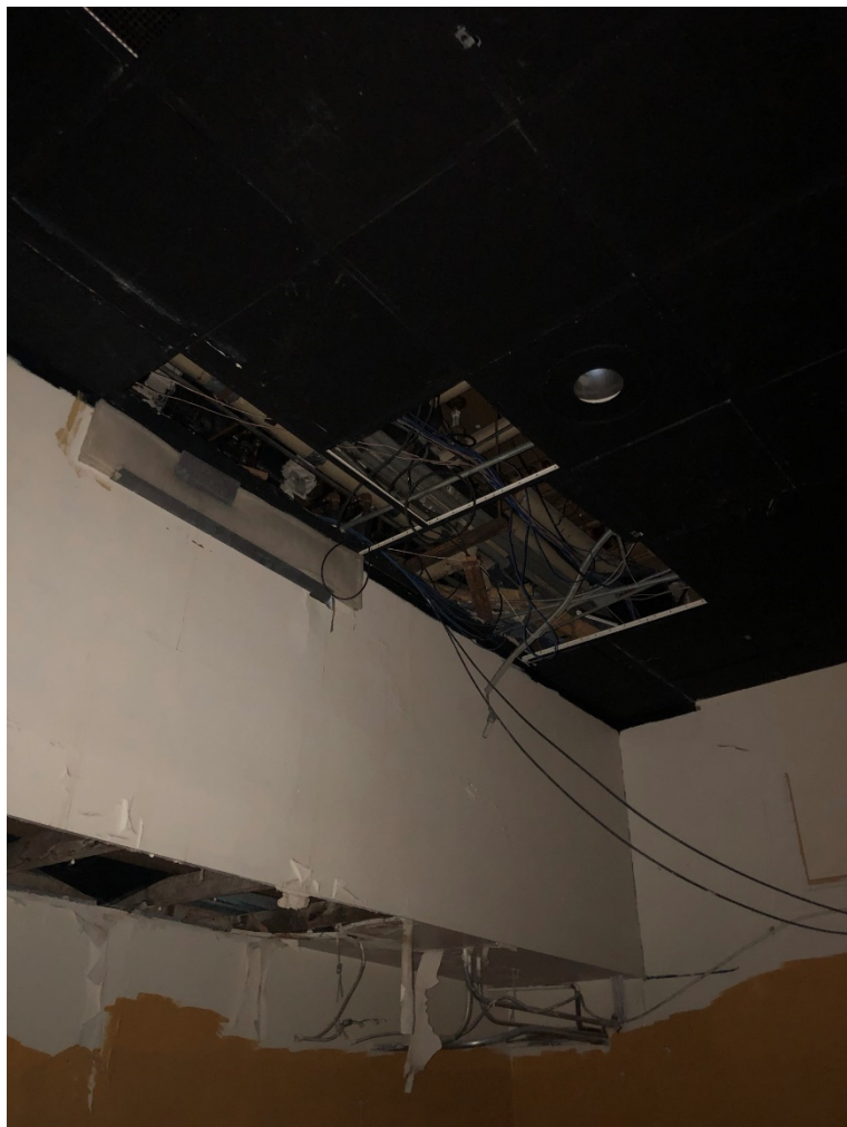
Photo OCH - 2 - 5: Room east of south lobby. Dropped ceiling covers original plaster ceiling. Original windows removed and openings blocked and covered.
