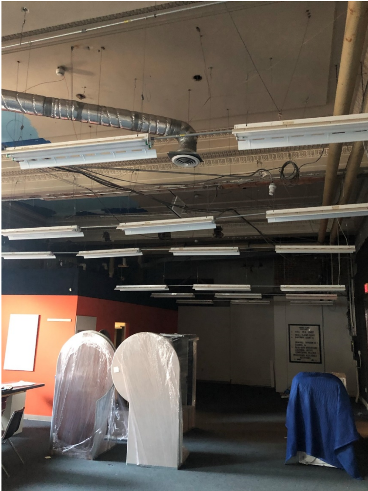
Photo OCH - 1 - 7: Room north of north lobby. Dropped ceiling removed. Exhibit walls in place. Same room as photos OCH-1-8 and OCH-1-9.
