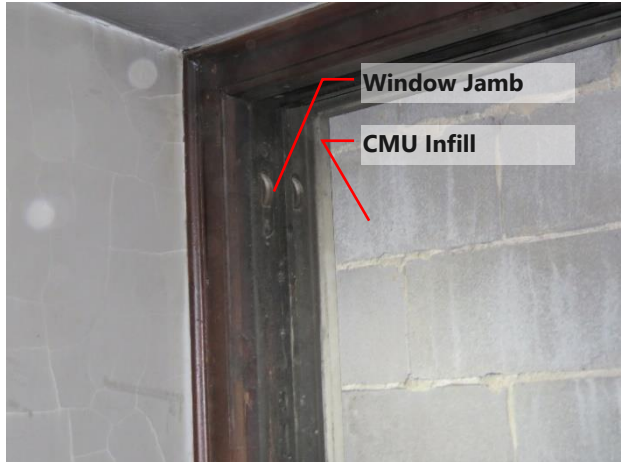
Figure 33. original wood window frame behind infilled window opening
