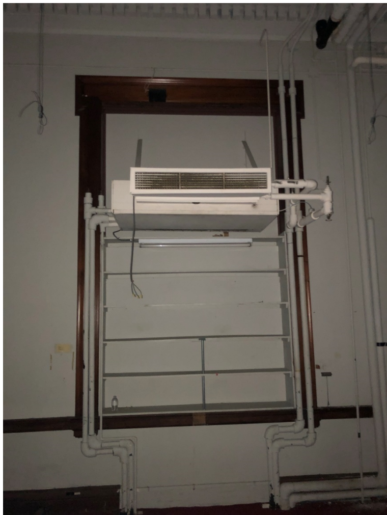
Photo OCH - 3 - 11: Room west of south lobby. Original window removed and opening blocked.
