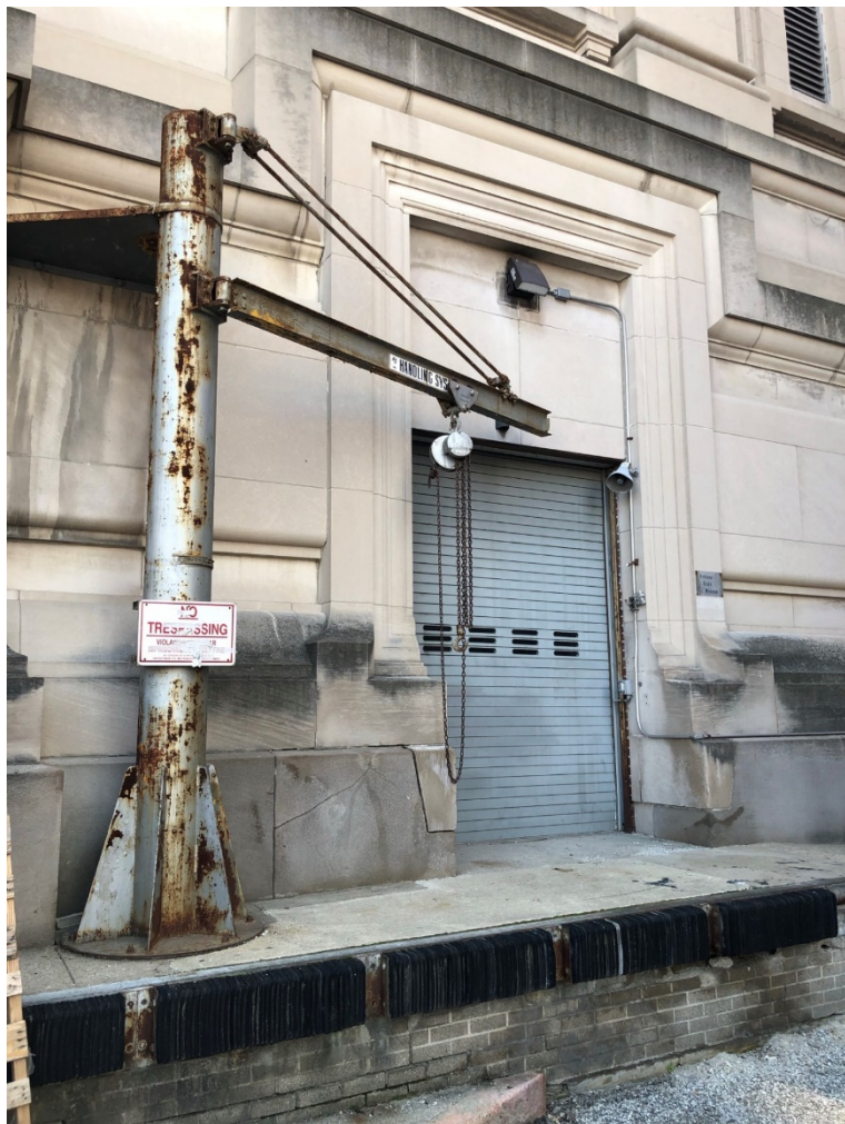
Photo OCH - EXT - 7: Loading dock and overhead door on west side adjacent to alley.
