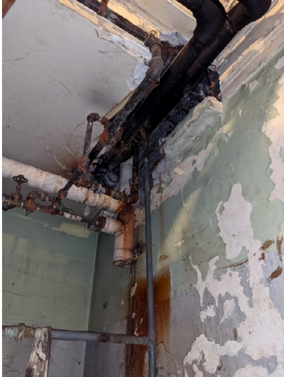
Figure 1 Existing Piping Chase – location basement northeast corner
