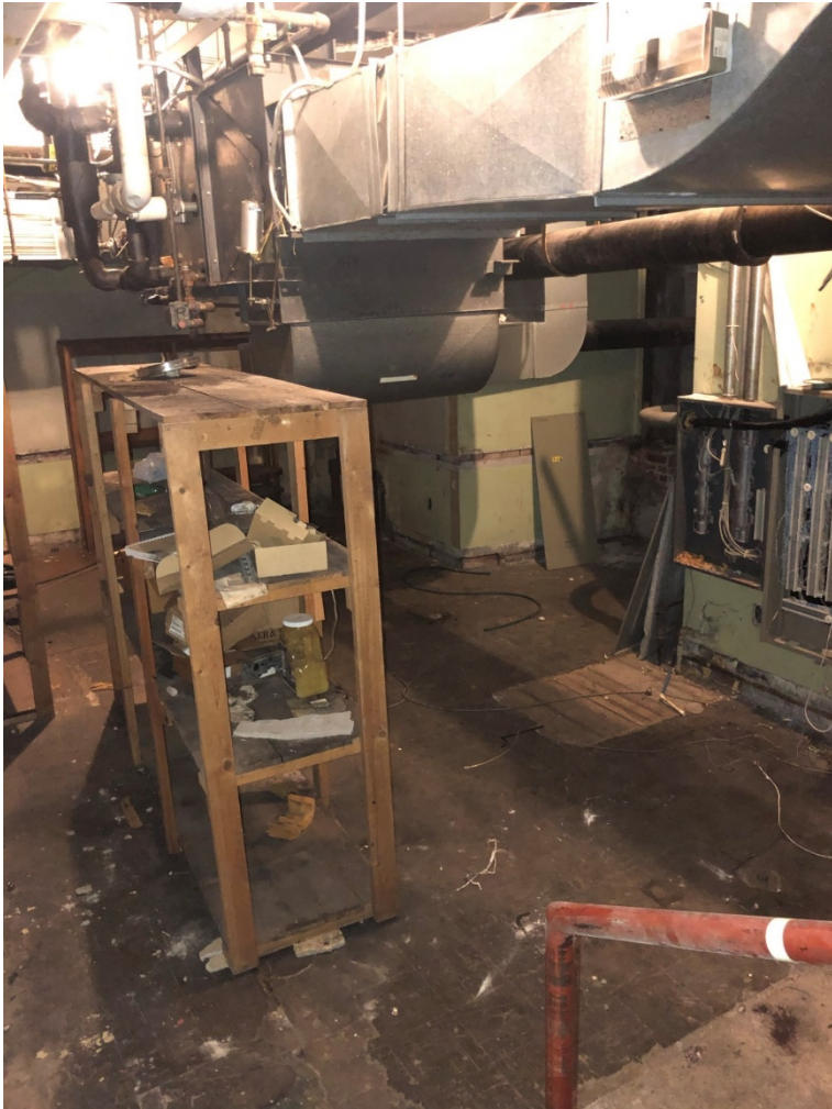
Photo OCH - B - 4: Mechanical room at west end of room south of south lobby.
