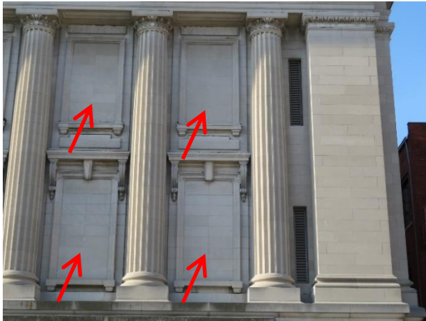
Figure 32. Infilled window openings on north facade.
