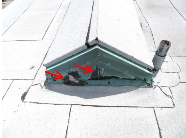
Figure 54. Liquid-applied repairs to copper flashings at small skylight on Roof Area 1.
