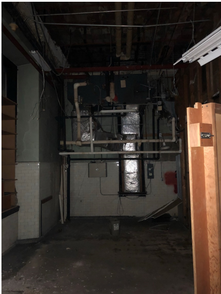
Photo OCH - 3 - 17: Divided space in room north of the north lobby. Original windows removed and blocked. Mechanical equipment serves the room north of the north lobby.
