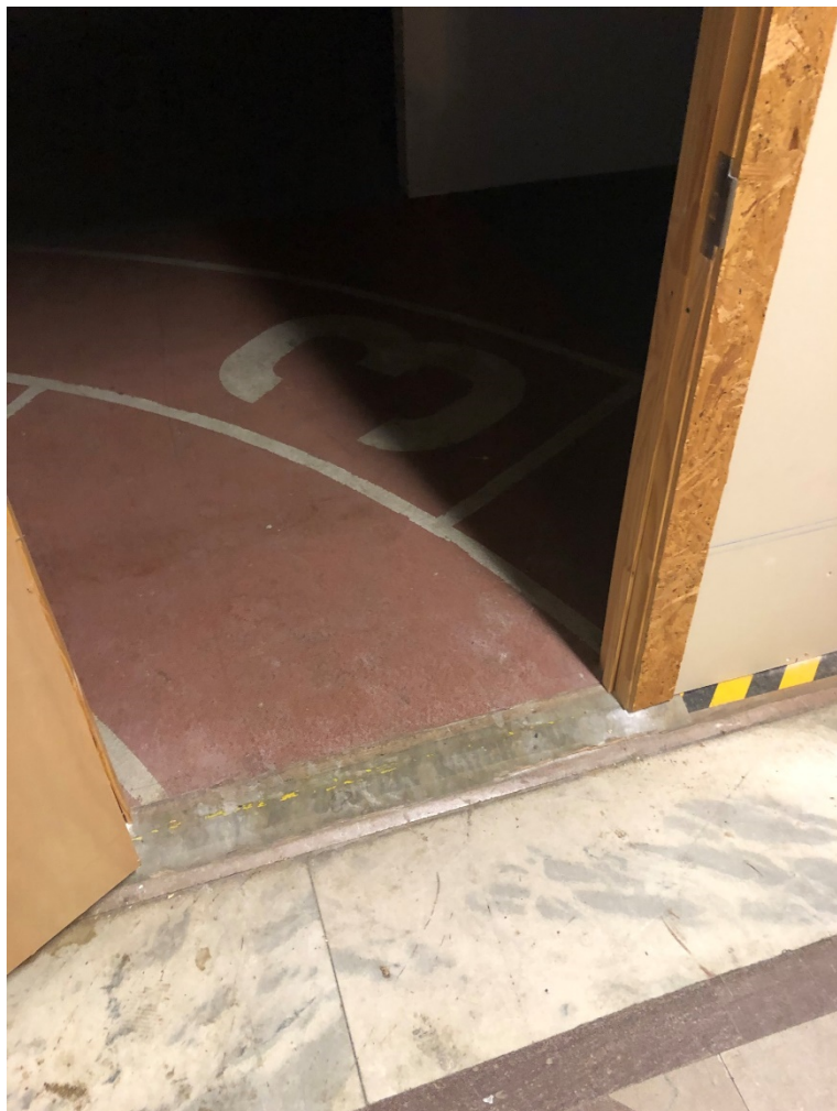
Photo OCH - 2 - 16: Non-original floor in room north of north lobby.
