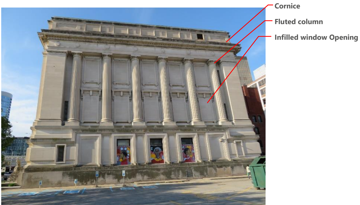
Figure 1. Overall view of the north facade.
