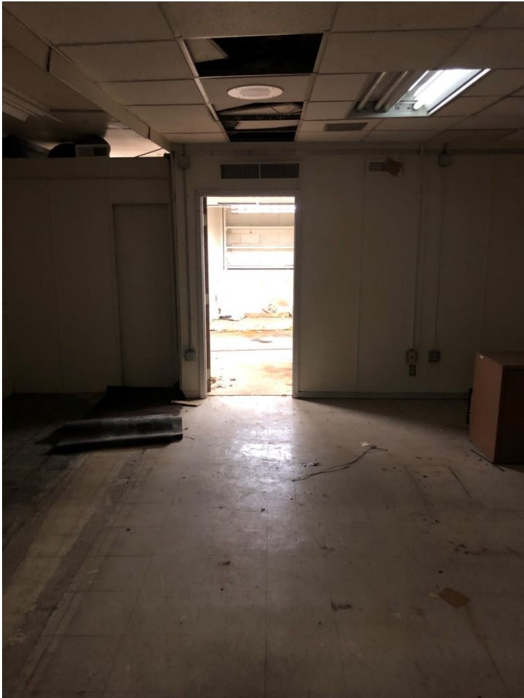
Photo OCH - B - 9: Room east of south lobby. Drop ceiling covers original ceiling. Same room as photo OCH-B-8.
