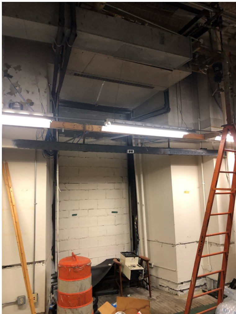
Photo OCH - 1 - 10: Room east of north lobby. Original window removed and opening blocked. Mechanical system up against ceiling.
