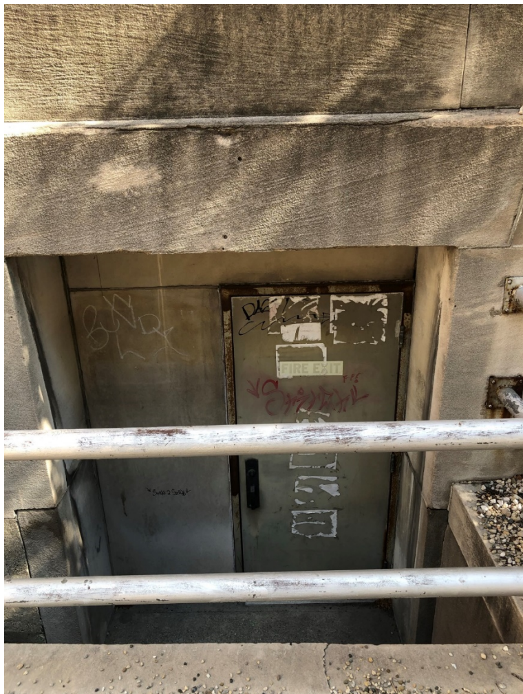
Photo OCH - EXT - 13: Basement egress door on south elevation adjacent to Ohio Street.
