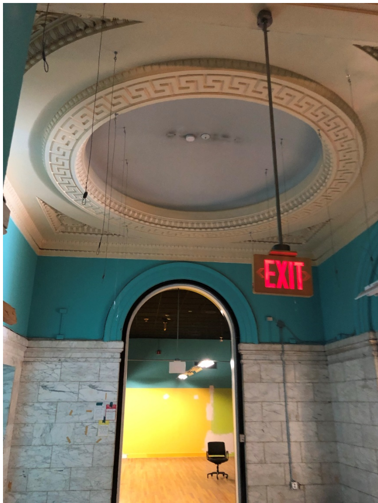
Photo OCH - 3 - 13: North lobby. Original plaster ceiling and wall and marblework largely intact.
