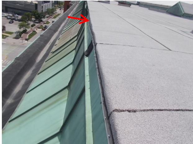
Figure 42. Edge metal termination of the mod-bit roof system.
