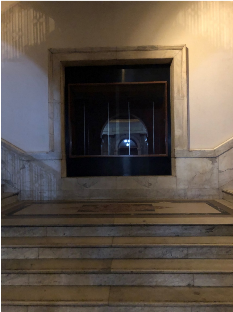
Photo OCH - 1 - 3: Landing at central stairs. Original window removed and blocked in. Used as display case.
