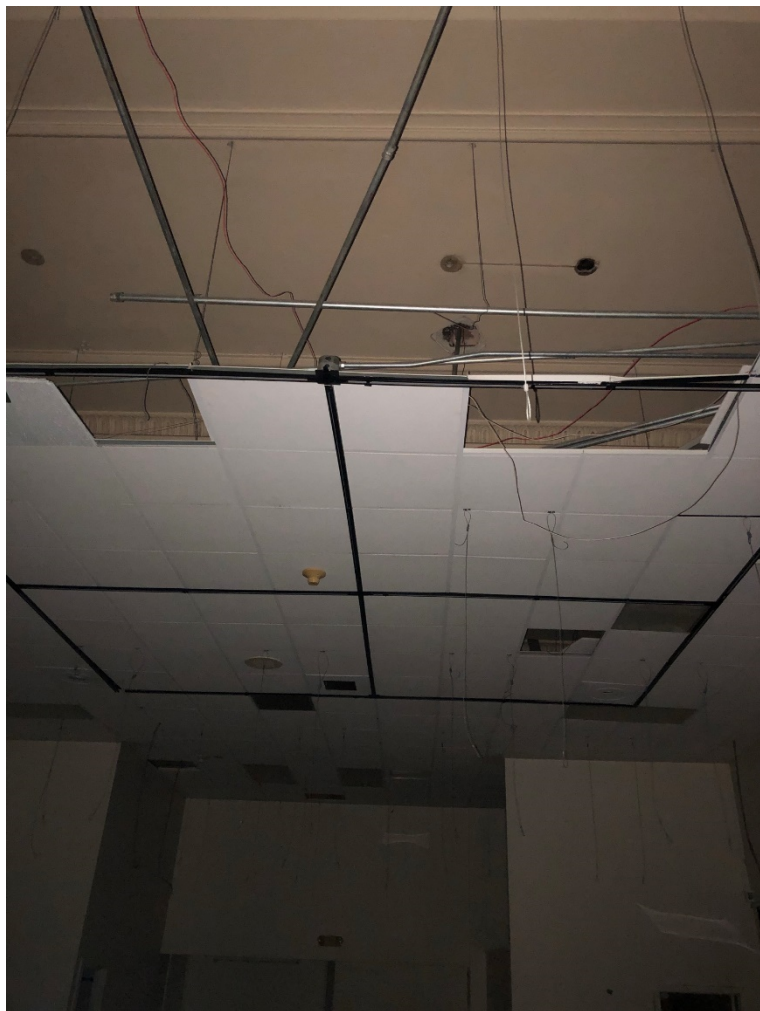
Photo OCH - 3 - 9: Room south of south lobby. Original plaster ceiling partially exposed. Plaster walls are not original and cover original walls. Same room as OCH-3-8 and OCH-3-10.
