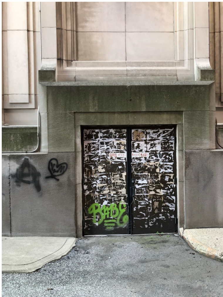
Photo OCH - EXT - 9: Egress doors at central stairs on west elevation adjacent to alley.
