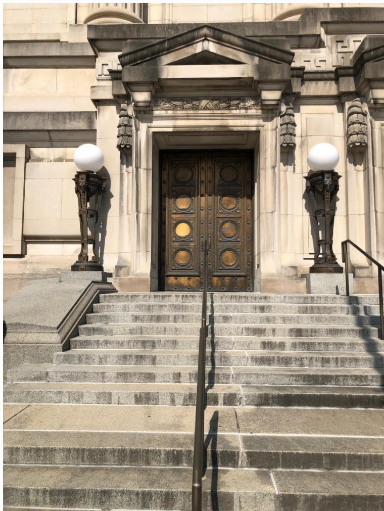
Photo OCH - EXT - 14: East elevation adjacent to Alabama Street. Stairs leading to bronze doors at vestibule.
