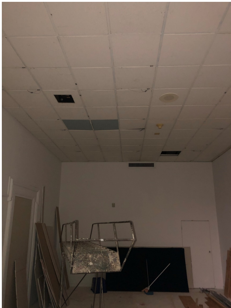
Photo OCH - 2 - 18: Room east of north lobby. Dropped ceiling covers original plaster ceiling. Plaster wall covers original plaster wall and blocked-in window opening.
