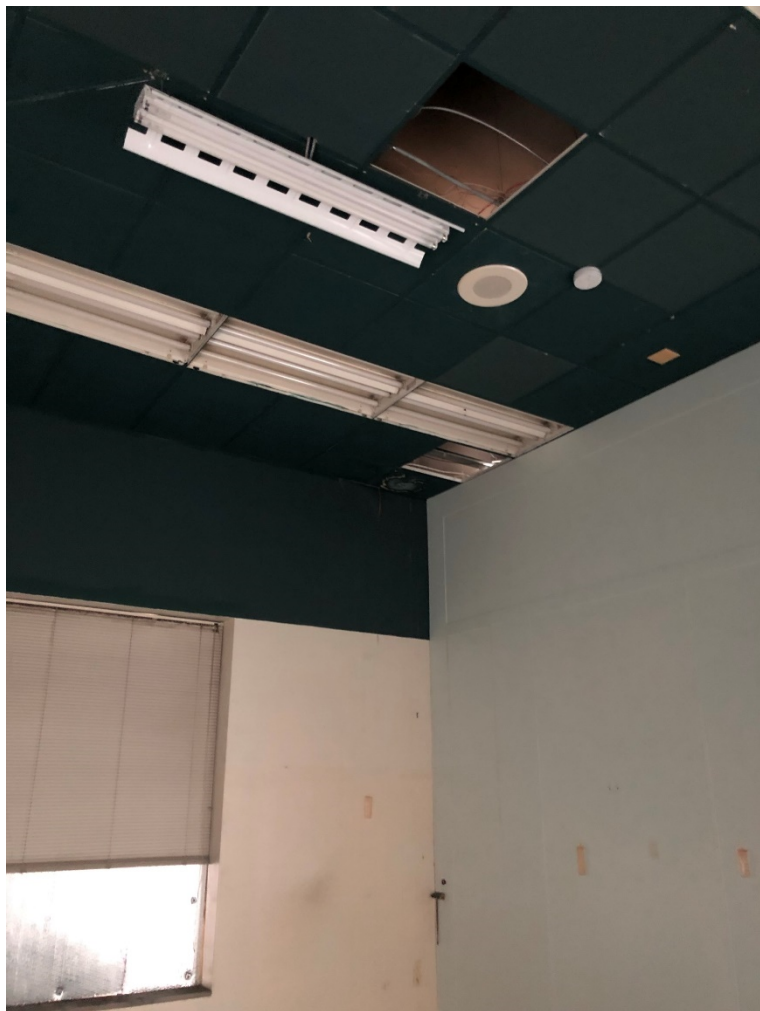
Photo OCH - 3 - 6: Room east of rotunda. Dropped ceiling covers original plaster ceiling. Windows are replacement and openings are partially blocked. Same room as Photos OCH-3-3 through OCH-3-5.
