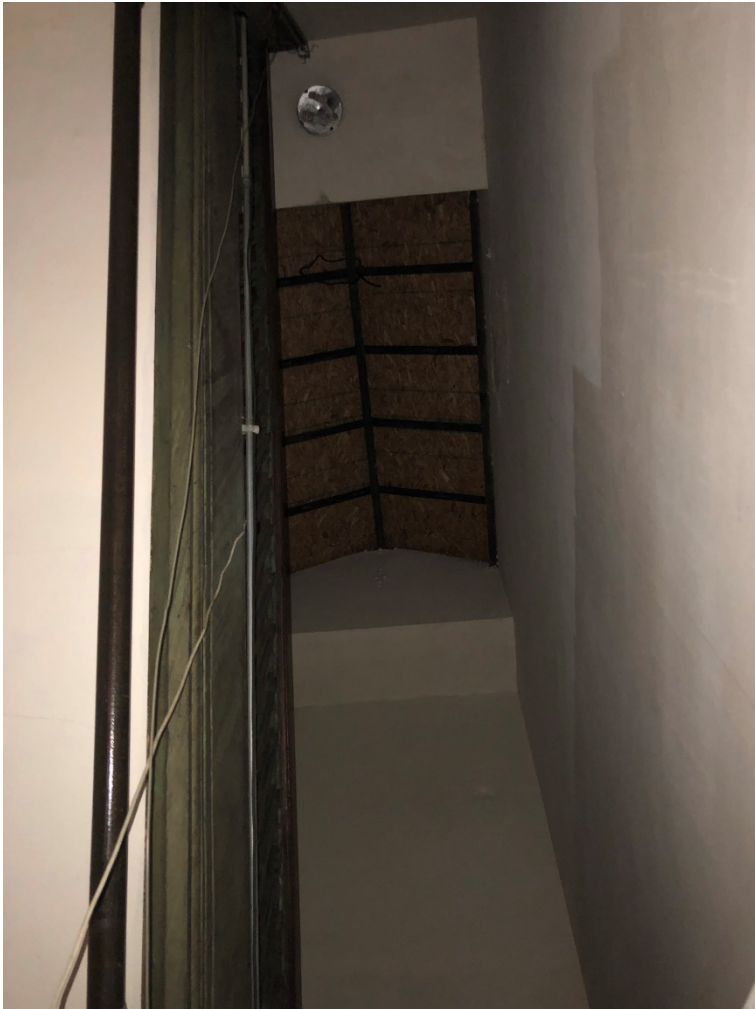
Photo OCH - 4 - 18: North private stair. Skylight over stairwell. Roofing installed over original skylight.
