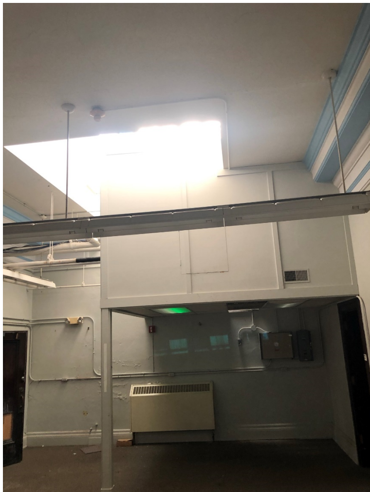
Photo OCH - 4 - 15: Office east of north lobby. Mechanical mezzanine partially covering skylight. Windows openings blocked in and plastered. Same room as OCH-4-16.
