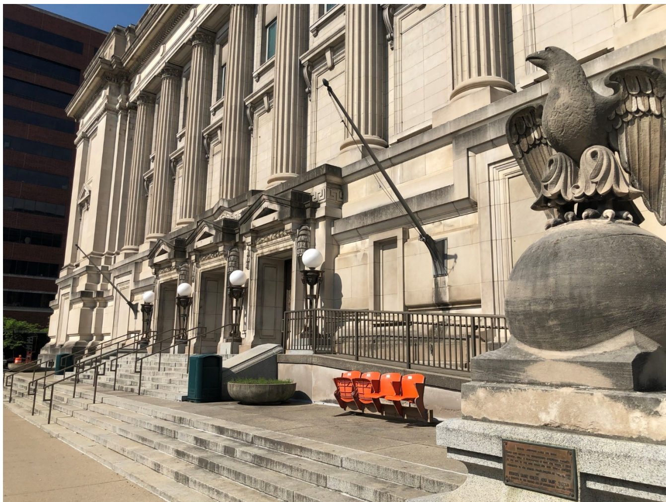
Photo OCH - EXT - 3: East/front elevation. Multiple original windows removed and openings blocked.
