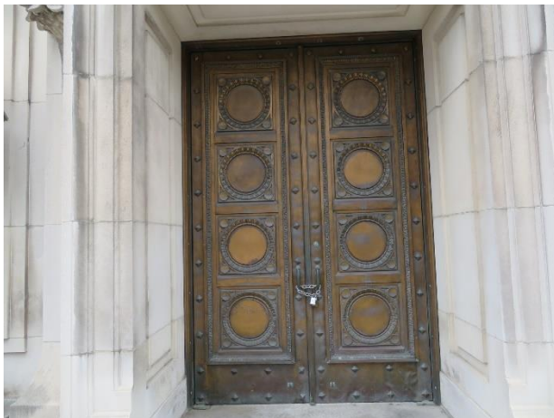
Figure 35. Overall view of one bronze clad door.
