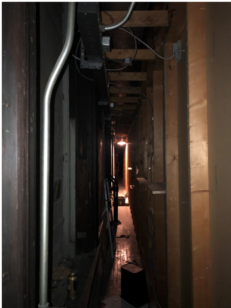
Photo OCH - 2 - 14: Room north of north lobby. Behind the exhibit walls.
