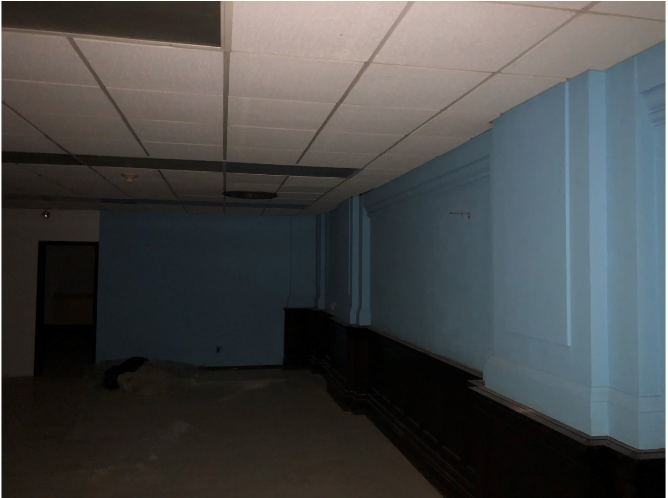
Photo OCH - 4 - 3: Council chamber. Drop ceiling covering original plaster ceiling. Window openings blocked in.
