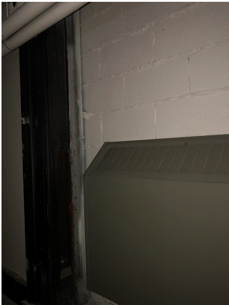
Photo OCH - 3 - 10: Room south of south lobby. Original windows removed and opening blocked. Same room as OCH-3-8 and OCH-3-9.
