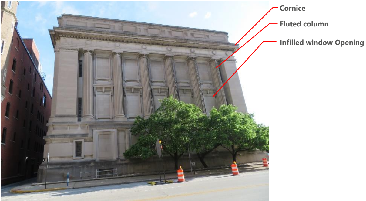
Figure 3. Overall view of the south facade.
