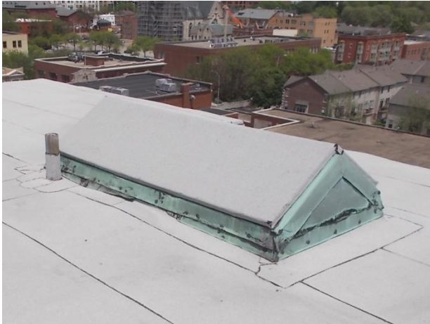
Figure 53. Skylight which has been covered with GSMB membrane.
