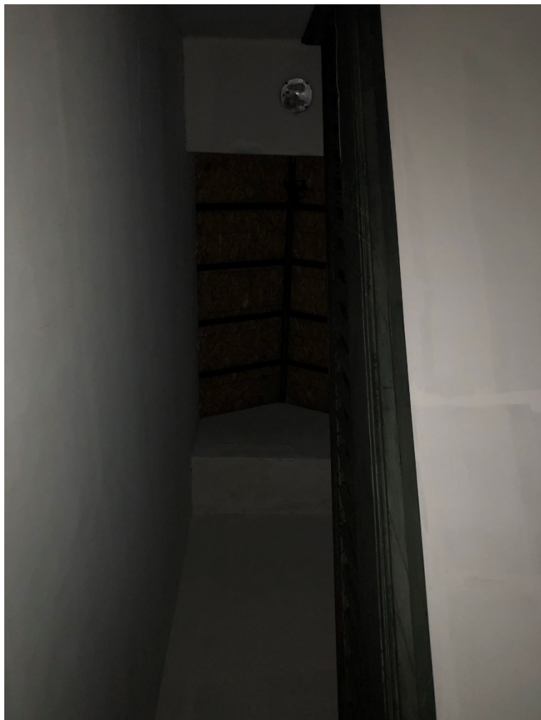
Photo OCH - 4 - 19: South private stair. Skylight over stairwell. Roofing installed over original skylight.
