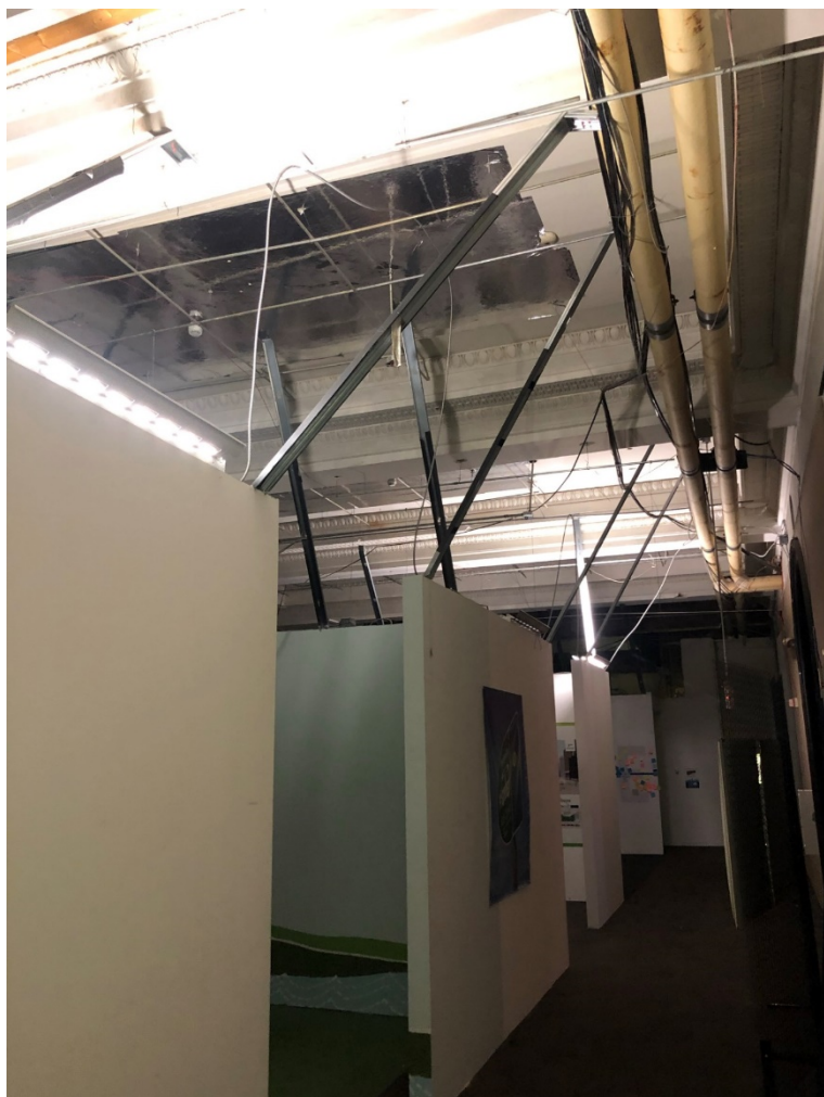
Photo OCH - 1 - 15: Room south of south lobby. Dropped ceiling removed. Exhibit walls in place. Same room as photo OCH-1-16.
