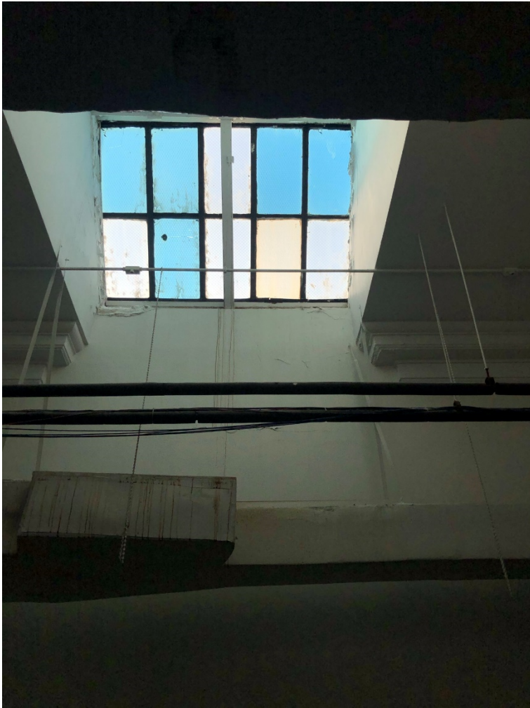
Photo OCH - 4 - 9: Office east of the rotunda. Original skylight. Same room as Photo OCH-4-8.
