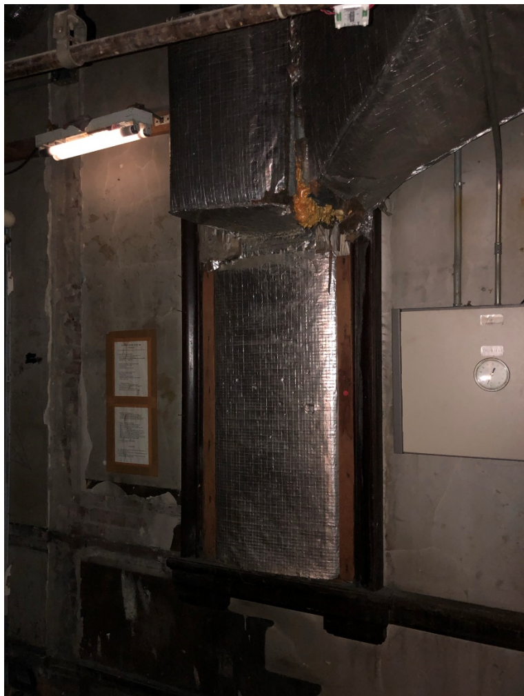
Photo OCH - 2 - 9: West end of room south of south lobby. Mechanical space located behind plaster exhibit walls. Original room removed and used for mechanical system. Same space as photos OCH-2-8 and OCH-2-10.
