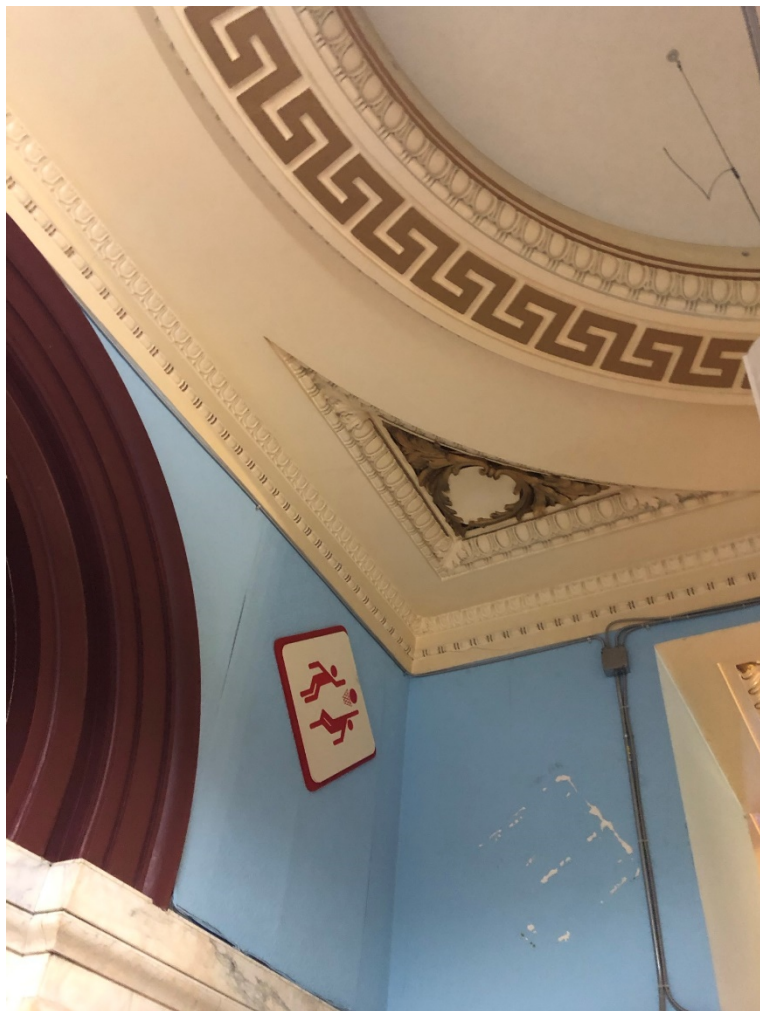
Photo OCH - 2 - 17: North lobby. Original plaster ceiling and walls. Exhibit graphics applied to original plaster.
