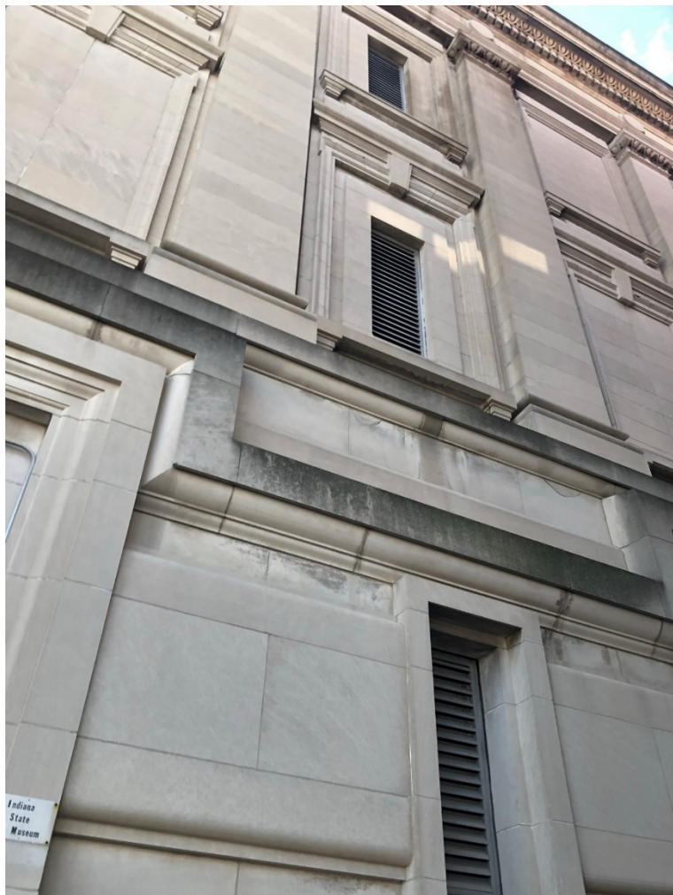
Photo OCH - EXT - 8: West elevation. Previous window openings at original bathroom locations.
