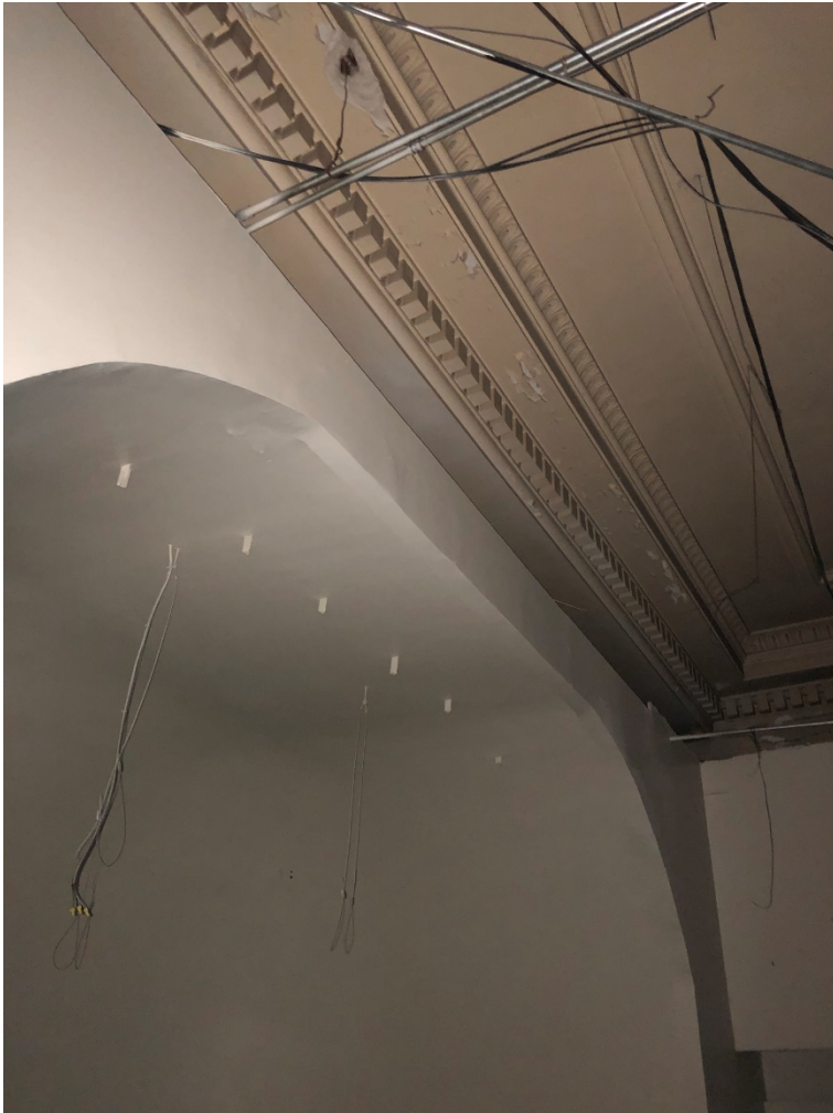
Photo OCH - 3 - 8: Room south of south lobby. Original plaster ceiling partially exposed. Plaster walls are not original and cover original walls. Same room as OCH-3-9 and OCH-3-10.
