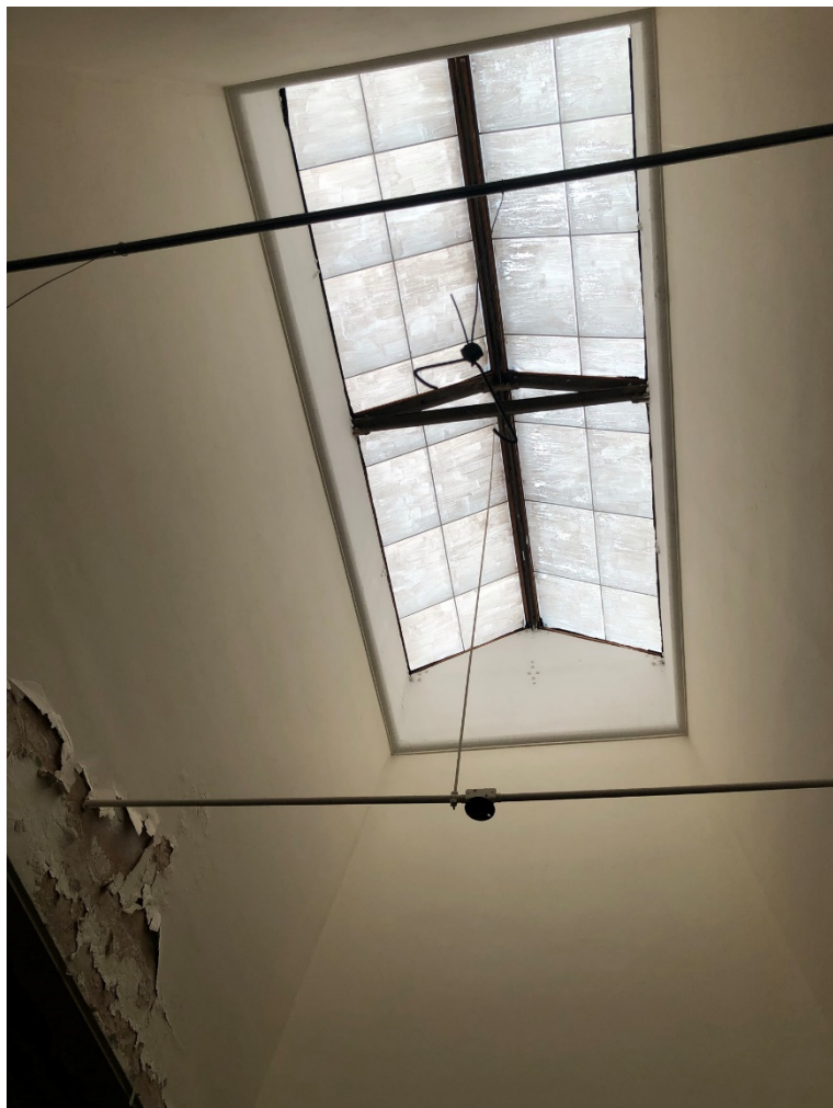
Photo OCH - 4 - 10: Lobby north of rotunda. Original skylight. Same room as Photo-OCH-4-11.
