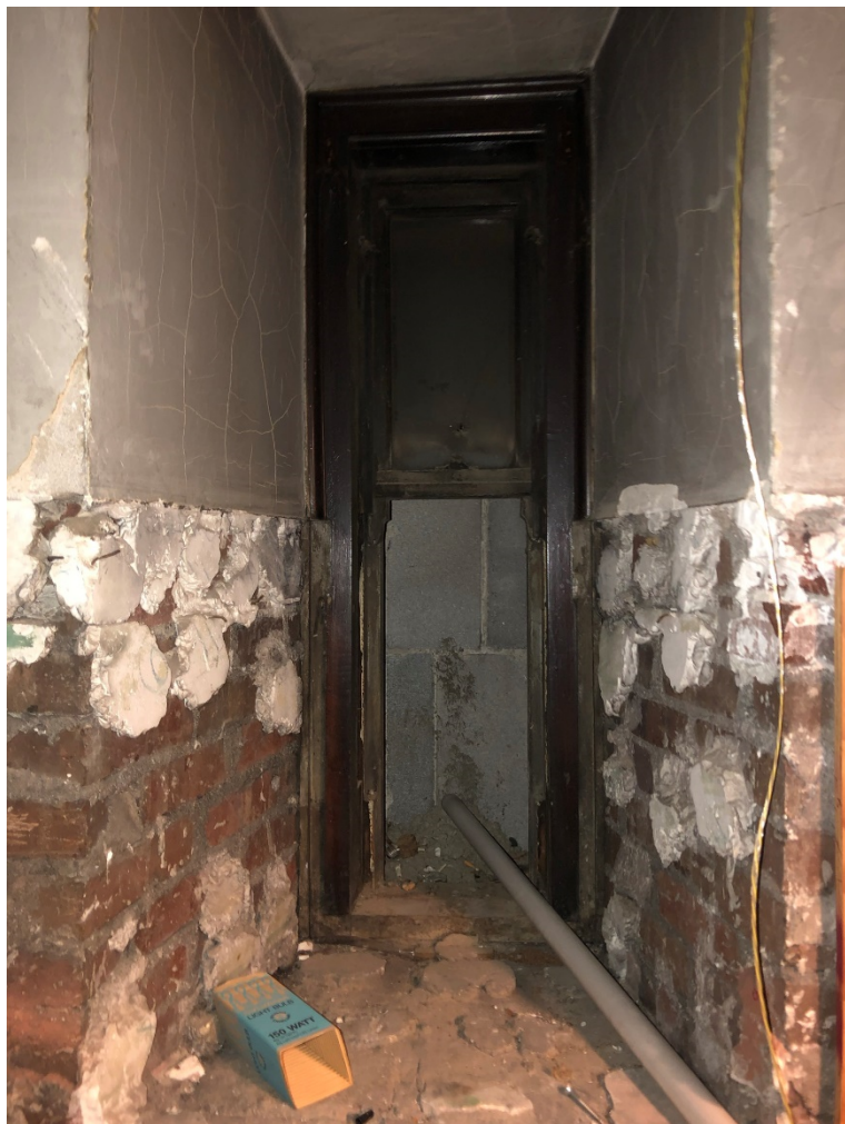
Photo OCH - 2 - 8: West end of room south of south lobby. Mechanical space located behind plaster exhibit walls. Original window removed and blocked in. Same space as photos OCH-2-9 and OCH-2-10.
