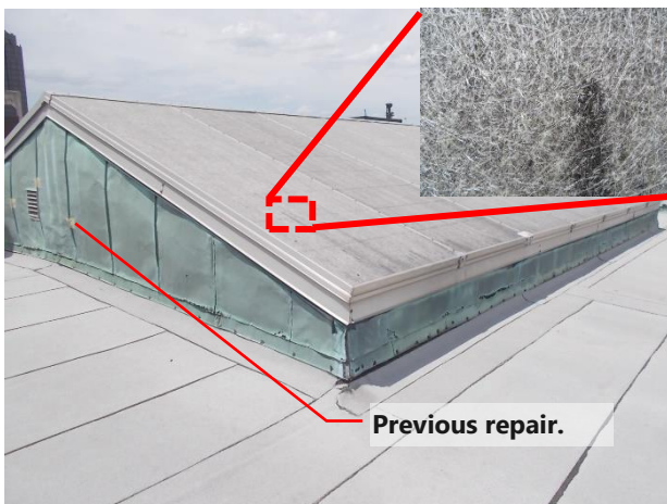
Figure 51. Atrium skylight with weathered fiberglass panels.
