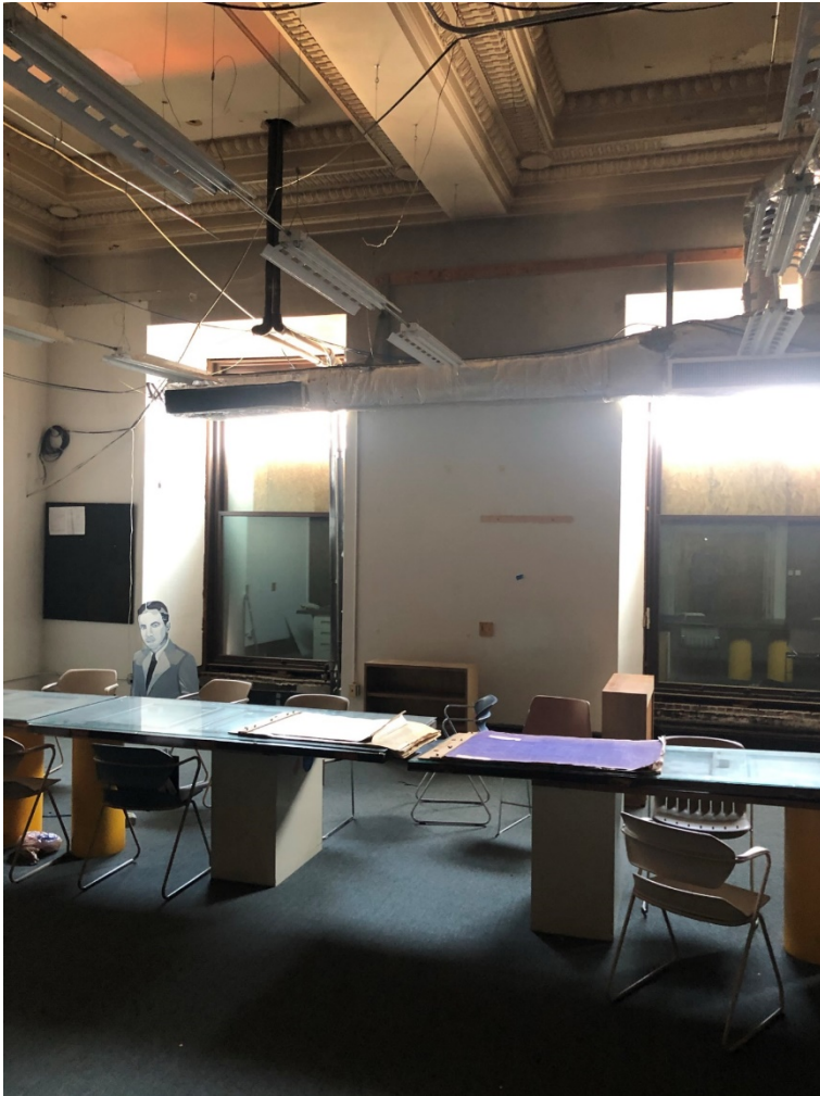
Photo OCH - 1 - 8: Room north of north lobby. Dropped ceiling removed. Three window openings restored. Same room as photos OCH-1-7 and OCH-1-9.
