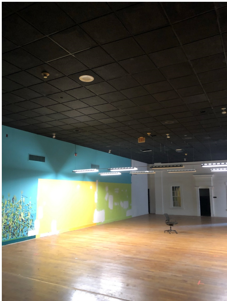
Photo OCH - 3 - 18: Room north of the north lobby. Dropped ceiling covers original plaster ceiling. Plaster walls are not original and cover original walls.
