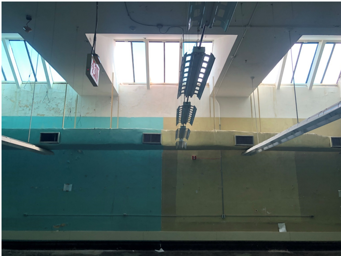
Photo OCH - 4 - 13: Office north of rotunda. Original plaster ceiling and skylights. Windows openings blocked in and plastered. Same room as OCH-4-14.
