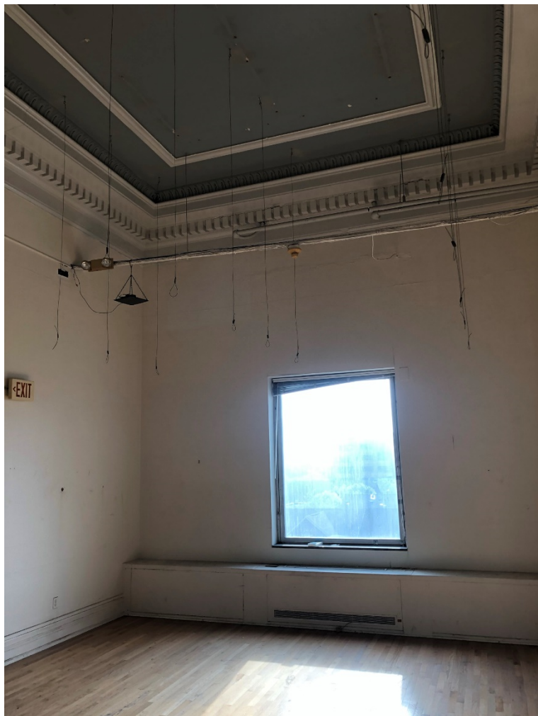
Photo OCH - 3 - 2: Room east of north lobby. Original ceiling intact. Window is replacement and opening is partially blocked.
