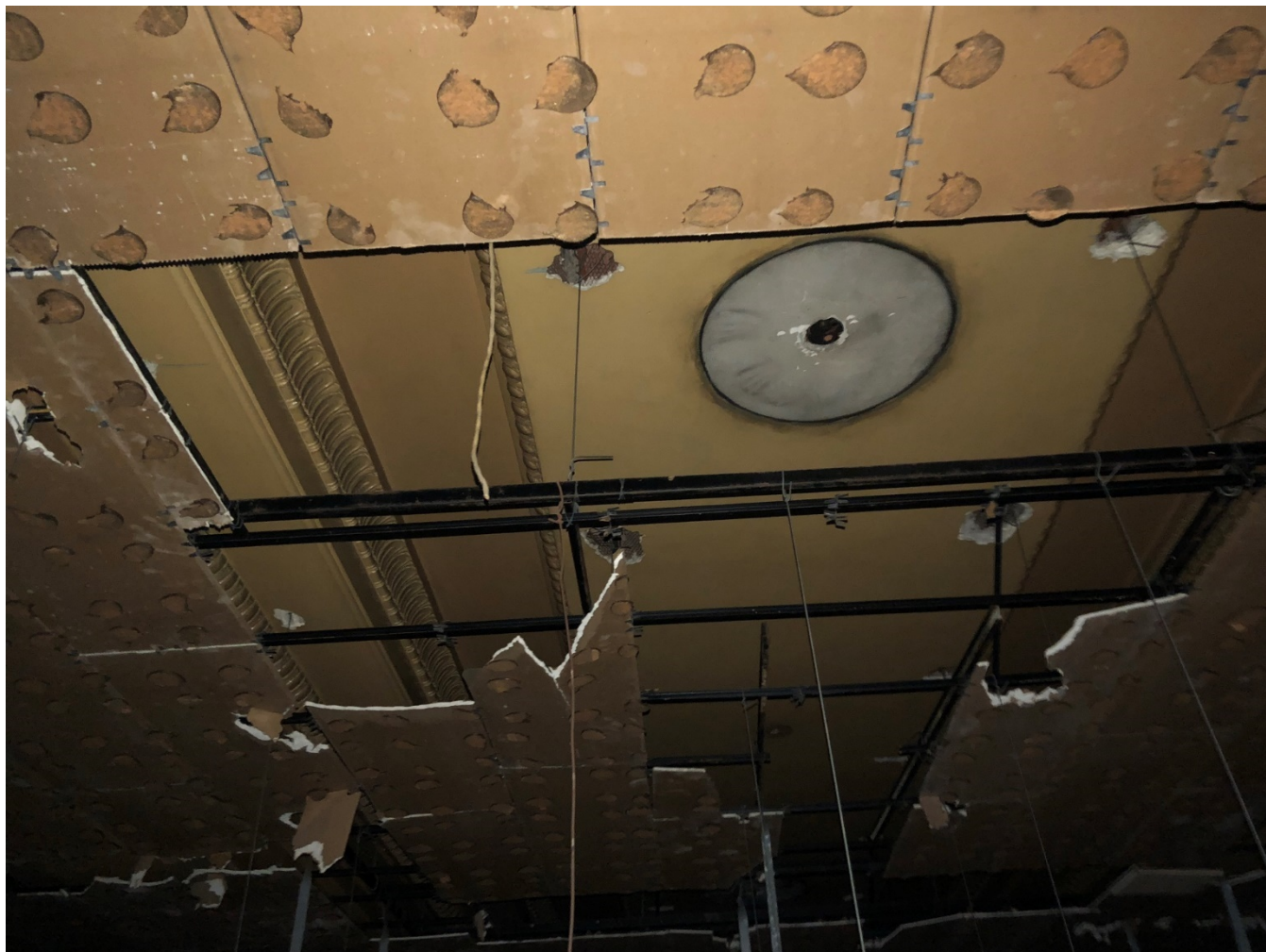
Photo OCH - 4 - 25: View from mezzanine looking at original plaster ceiling.
