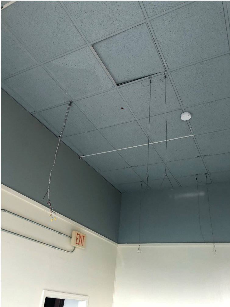
Photo OCH - 3 - 4: Room east of rotunda. Dropped ceiling covers original plaster ceiling. Windows are replacement and openings are partially blocked. Same room as Photos OCH-3-3 through OCH-3-6.
