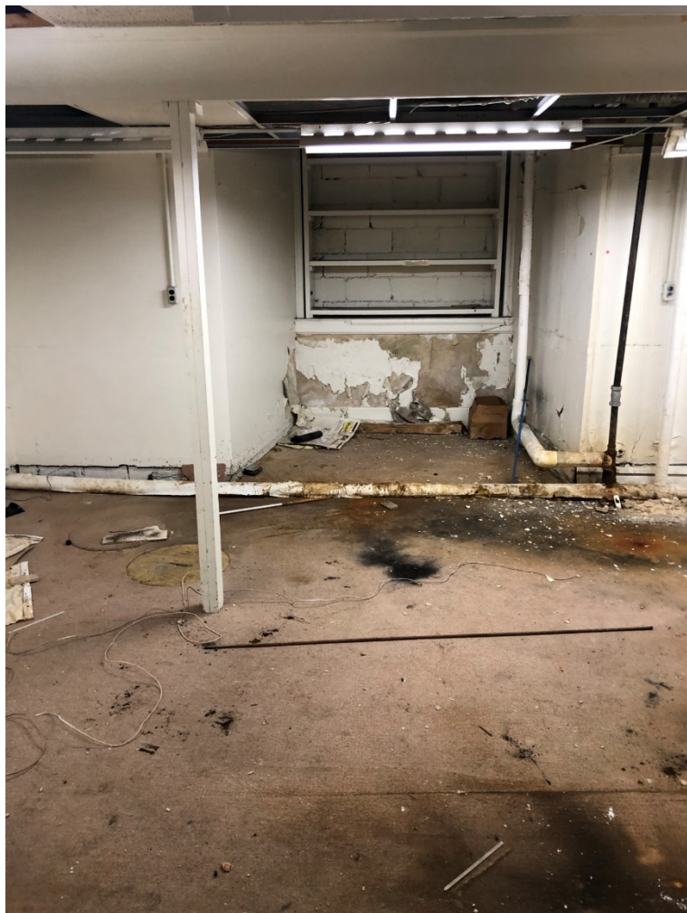
Photo OCH - B - 8: Room east of south lobby. Same room as photo OCH-B-9.
