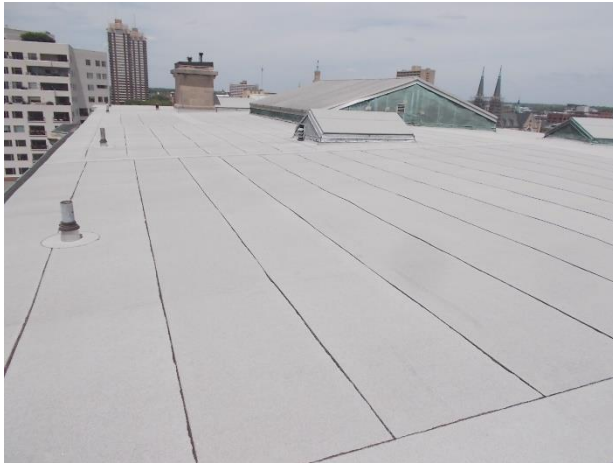
Figure 41. Overall view of Roof Area 1 showing atrium skylight and two small skylights.
