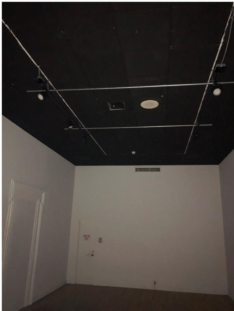
Photo OCH - 2 - 11: Room west of south lobby. Dropped ceiling covers original plaster ceiling. Plaster wall covers original plaster wall and blocked-in window opening.
