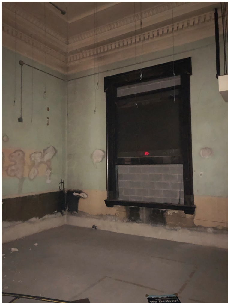
Photo OCH - 3 - 16: Room west of north lobby. Original window removed and blocked. Adjacent to freight elevator.
