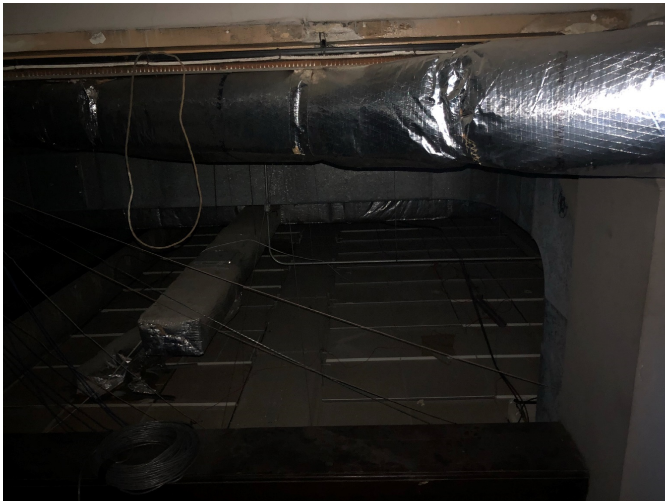
Photo OCH - 4 - 24: View from mezzanine looking over council chambers. Suspended ceiling blocks view. Ductwork fills space about suspended ceiling.
