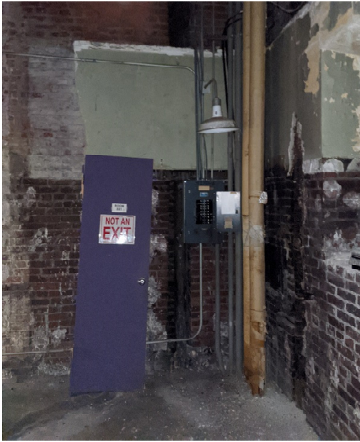
Figure 3 Piping Riser – location northwest corner fourth floor
